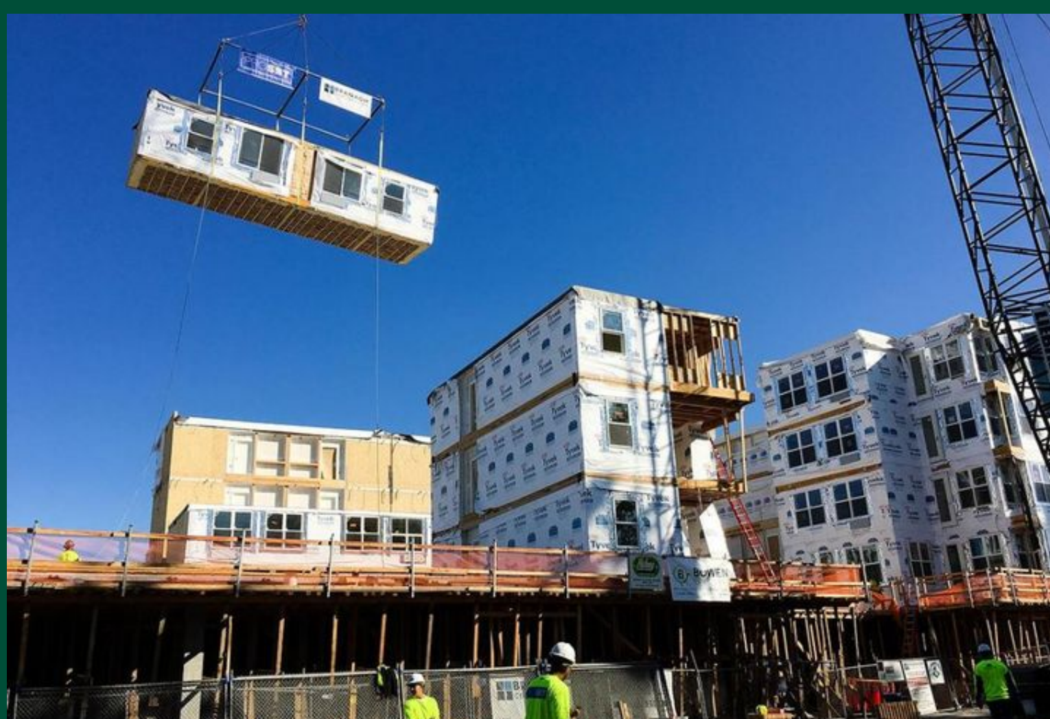
Figure 1: Onsite Installation for Modular construction .
